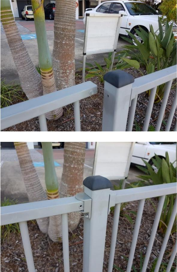
The top photograph shows a white pool fence panel with a missing bracket at its connection point to a post. The bottom photograph shows the same panel after the bracket has been replaced, ensuring a secure connection. |
